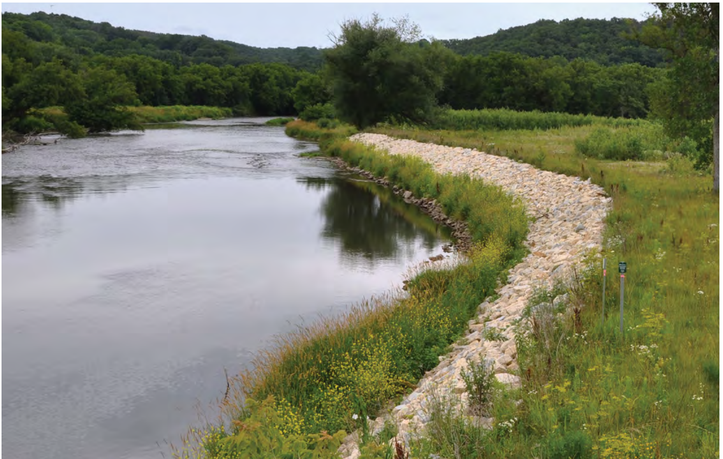
Streambank stabilization. Photo courtesy of Jason Johnson, USDA Natural Resources Conservation Service.
